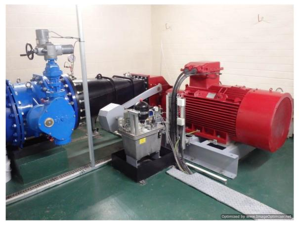
Figure 4: CINK Crossflow Turbine with directly-coupled 100 kW generator (Hydromatch Ltd)
