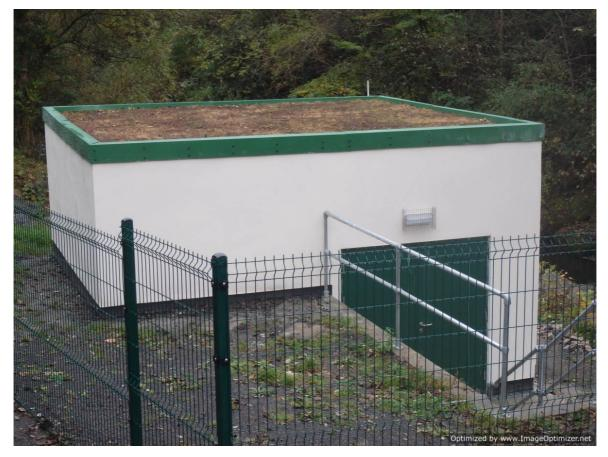
Figure 6: Taff Bargoed Hydropower scheme. A secure building of area approximately 5 x 5 m is required to house the hydropower equipment. The construction needs to consider future access for maintenance and comply with local planning preferences. The construction will influence whether operation of the equipment is audible from the outside.
