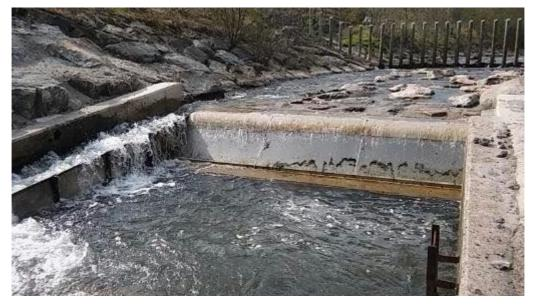
Figure 5: Conada type intake screen with fish pass flume alongside. Water is ducted from a sump beneath the screen via a low pressure pipe to a deeper chamber further into the bank where the water level sensor and penstock pipe are connected.
